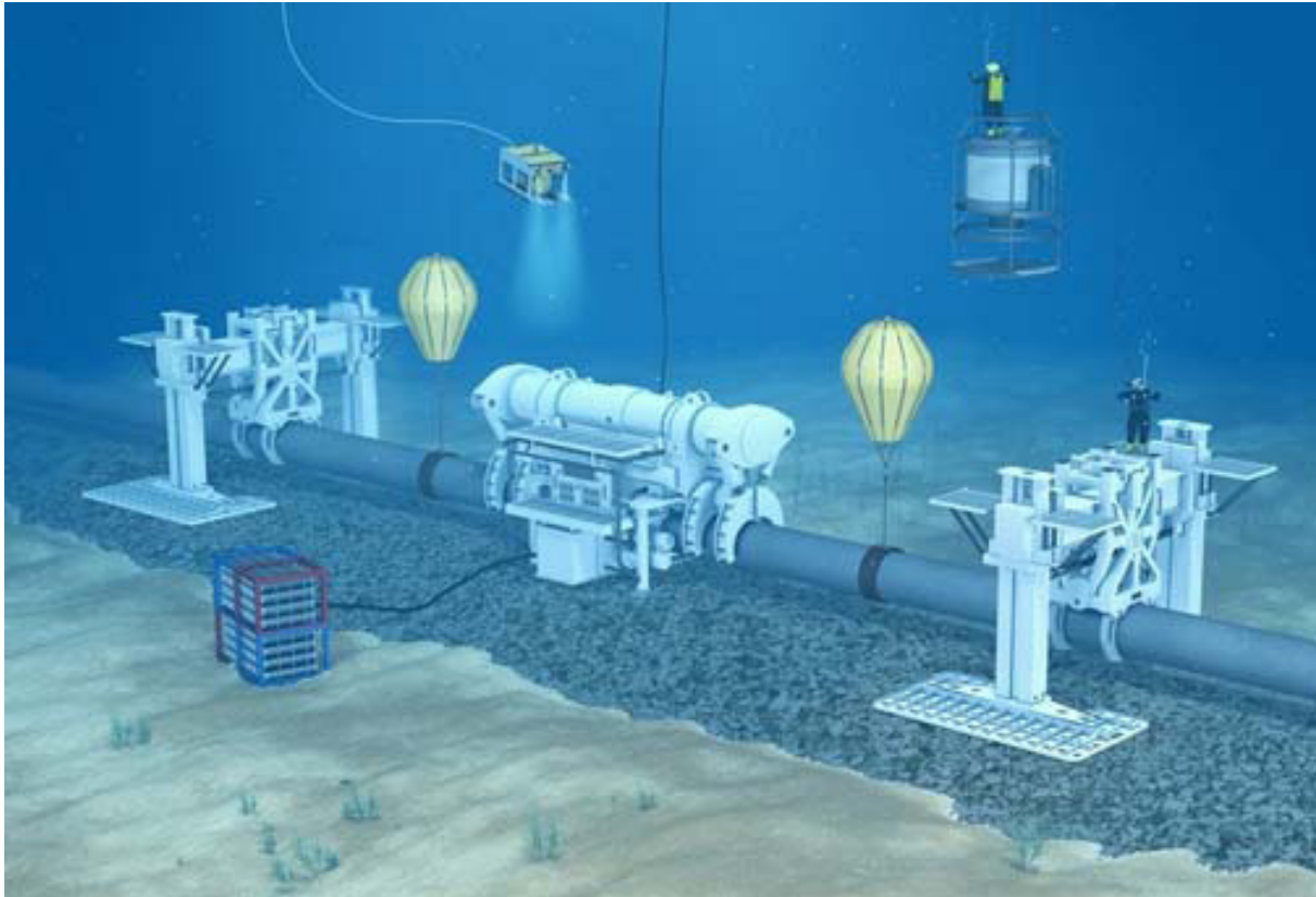
Figure 5.5 Hyperbaric tie-in set-up.
