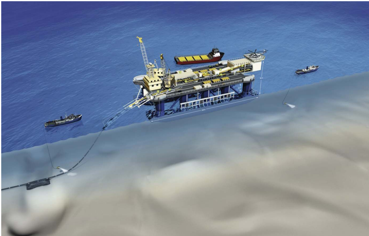
Figure 5.4 The S-lay pipe-lay vessel and survey support vessels.
